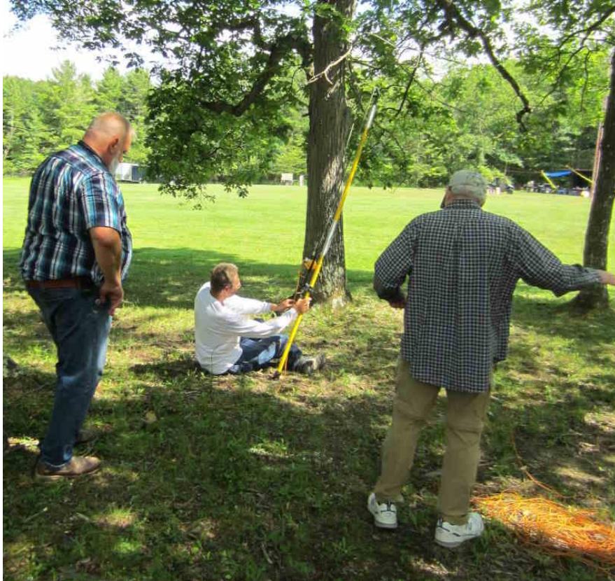
Fred K2TR Uses a Slingshot to Set a Wire Antenna
